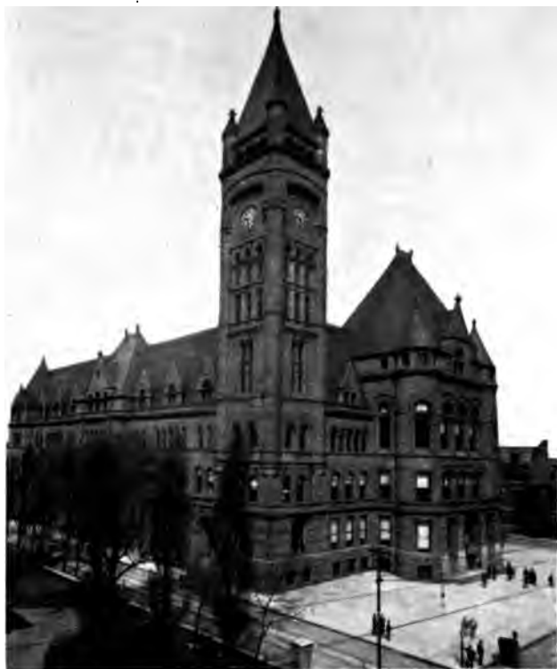
B. HANNAFORD & SONS, ARCHITECTS CITY HALL, CINCINNATI.
